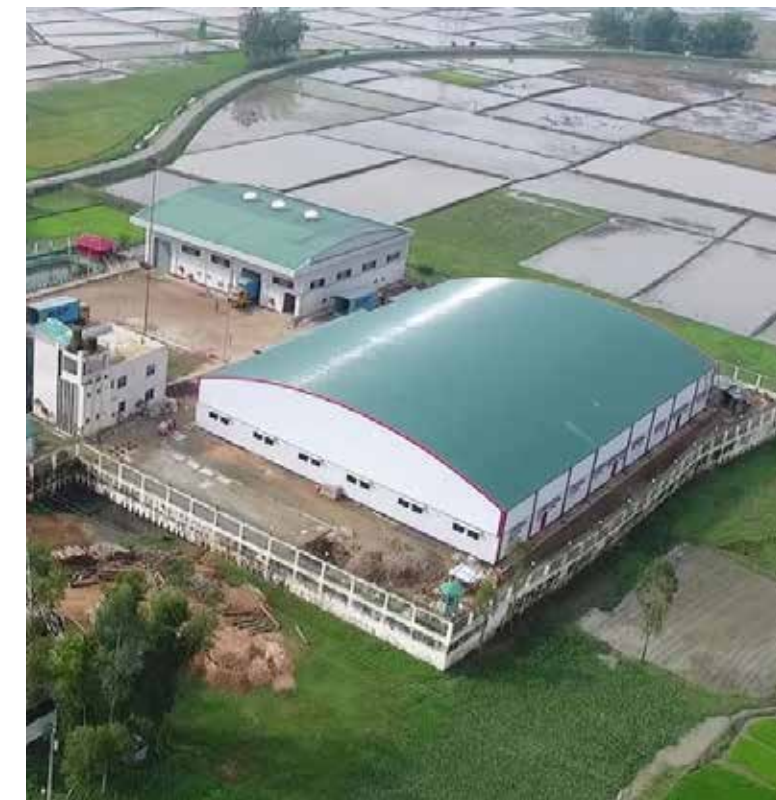
Aerial greener view of Sayestaganj warehouse
