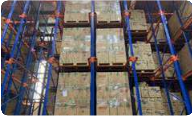
Vertical expansion- Rack installation
