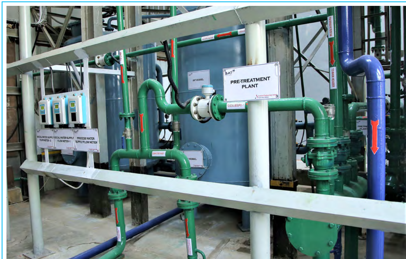
■ Water Line Re-networking at GLTP
